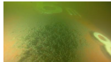
Coating adhesion failure
