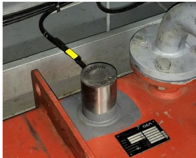
Fig.5: Ultrasonic transducer, source: Hasytec
