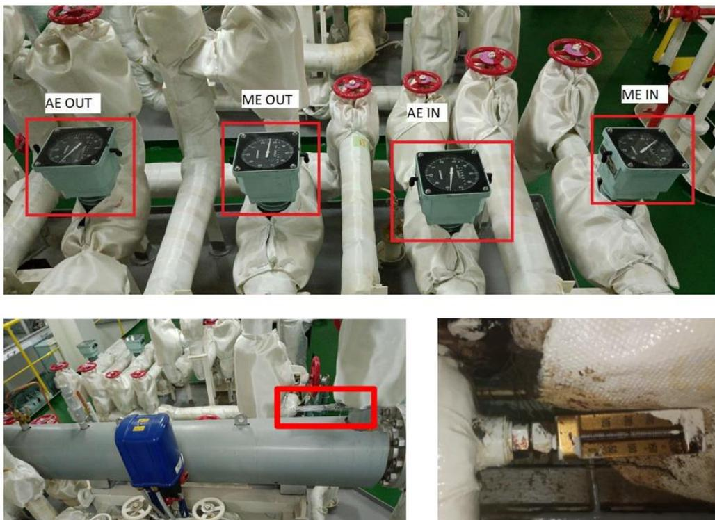
Fig. 4: Examples of onboard analogue volumetric flowmeters and FO thermometers
