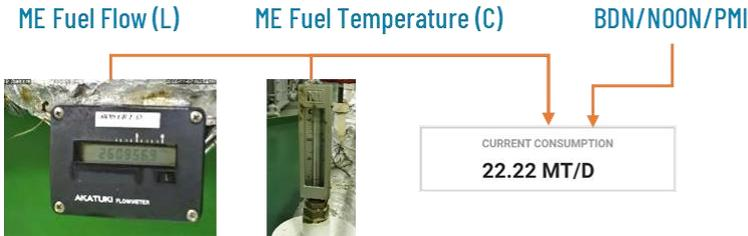
Fig.6: Mass flow calculations from volumetric flow, temperature, and FO parameters
