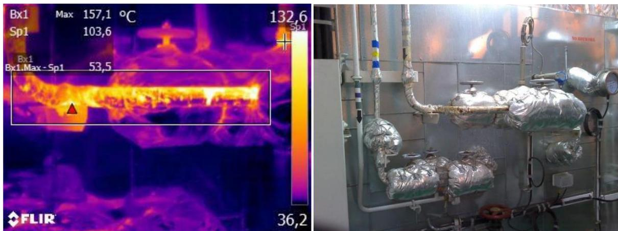
Fig.10: Thermally pictures of non-insulated fuel oil system
