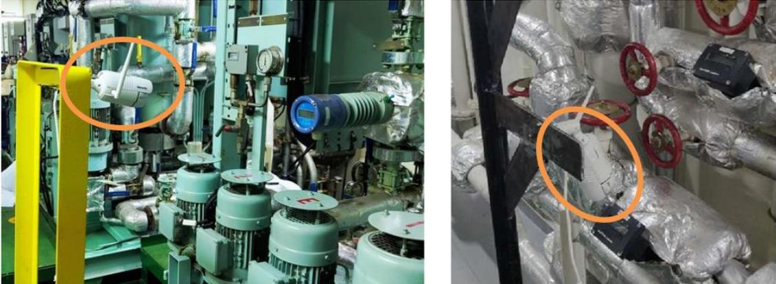
Fig.5: Positioning of cameras for consumption monitoring
